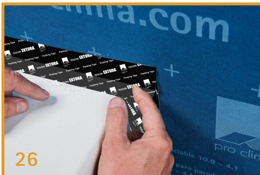
TESCON EXTORA® Pressure sensitive adhesive tape for overlaps and end laps in SOLITEX EXTASANA® system.
